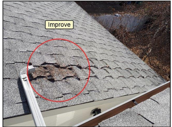
11. Discharging onto roof
