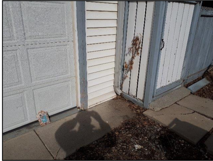
9. Downspouts end too close to building
