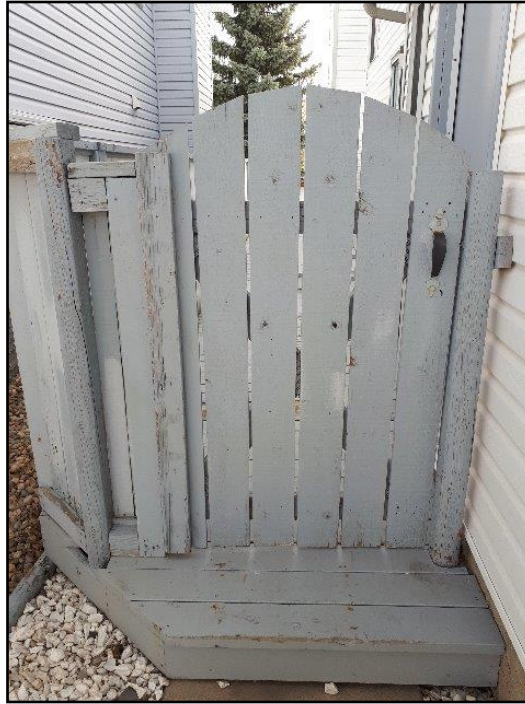
18. Gate - adjustment needed
