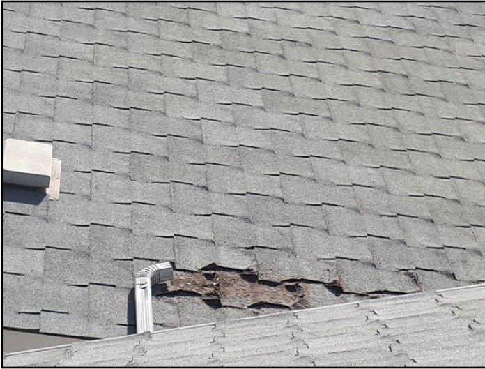
10. Discharging onto roof
