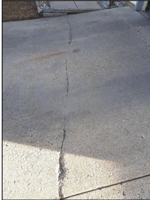
15. Cracked or damaged surfaces
