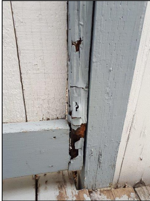
17. Boards damaged
